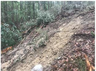
Looking across gully slope to south of proposed embankment dam wall. Silty sand soils exposed overlying weathered rock.
